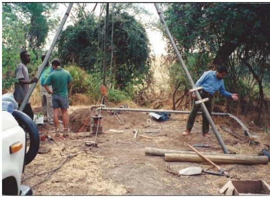
Bore hole drilling by Chobe River
